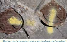
Drains and openings were spot-welded and marked
